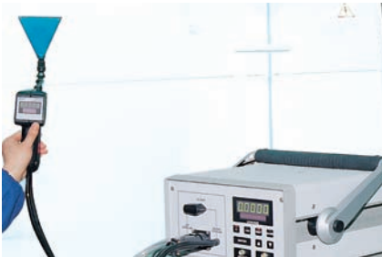
Integrity testing of HEPA filters
